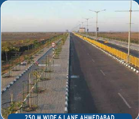
250 M WIDE 6 LANE AHMEDABAD -DHOHLERA EXPRESS WAY
