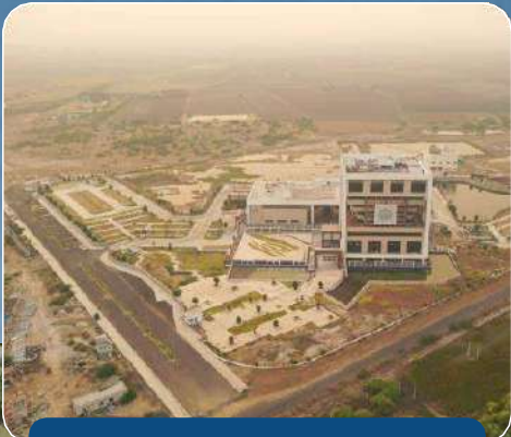
DHOHLERA ABCD BUILDING
